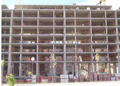
Figure 1: Typical building structure with reinforced concrete members.
